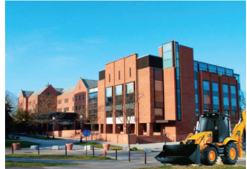
A preview of the construction set to begin this winter. Cost estimates and the sources of funding, have not yet been released as public information. Raether's updates may indeed just be elaborate money laundering.
