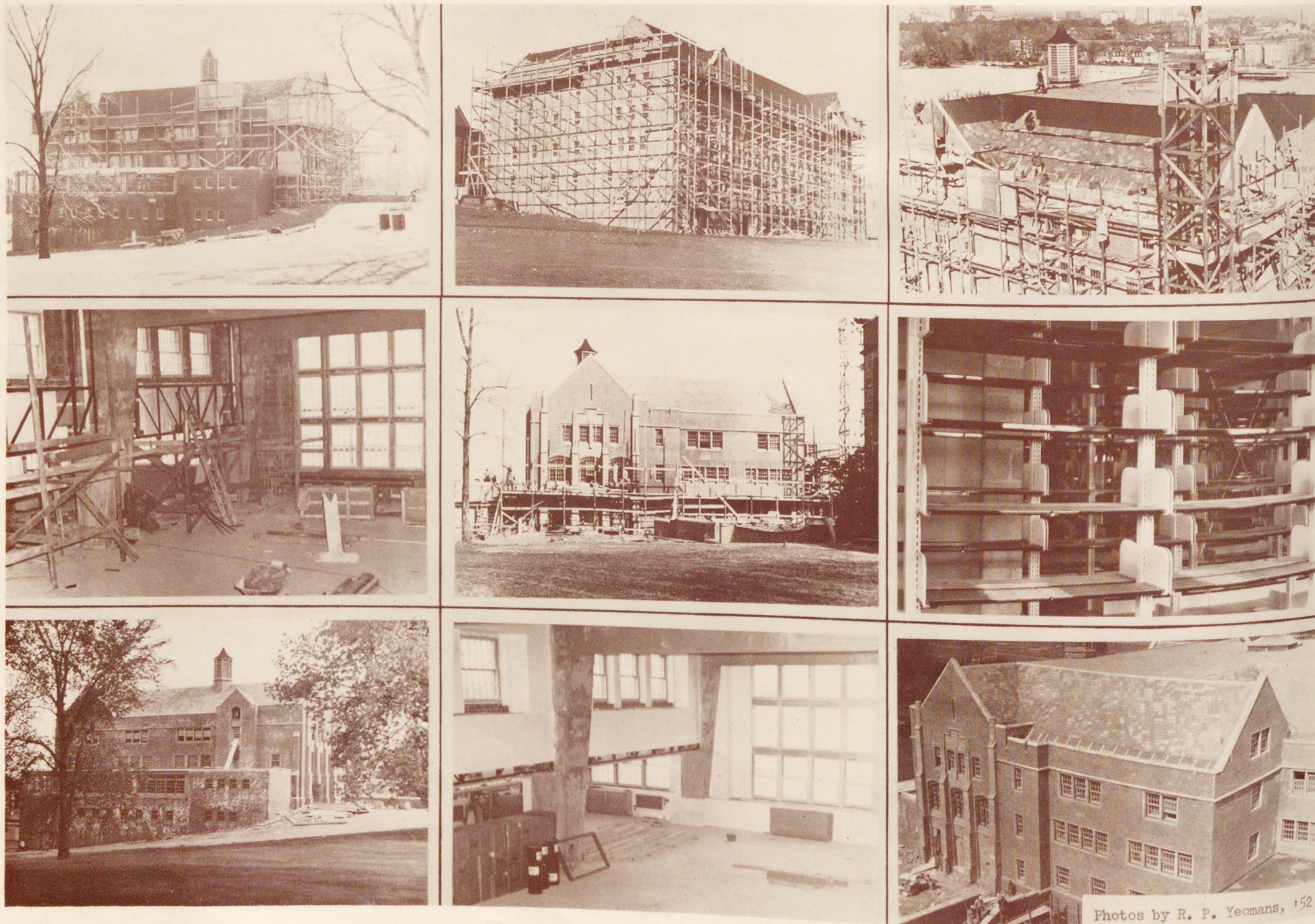
Top: Feb. 6, 1952—The building nears its final form; Feb. 6—A view of the southeast corner; Feb. 29—The slate roof is nailed on. Second row: Mar. 20—The reading room again, this time enclosed and dry; Apr. 11—Final cleaning and finishing of the main entrance; May 9—A portion of the 25 tons of stacks in the new library. Bottom: May 9—Leaves on the trees again and complete except for cleaning and finishing touches; May 9—Decorating of the reading room begins; May 9—A little paint on the windows and landscaping and the job is done. (All photos in this series by Richard P. Yeomans, '52.)
