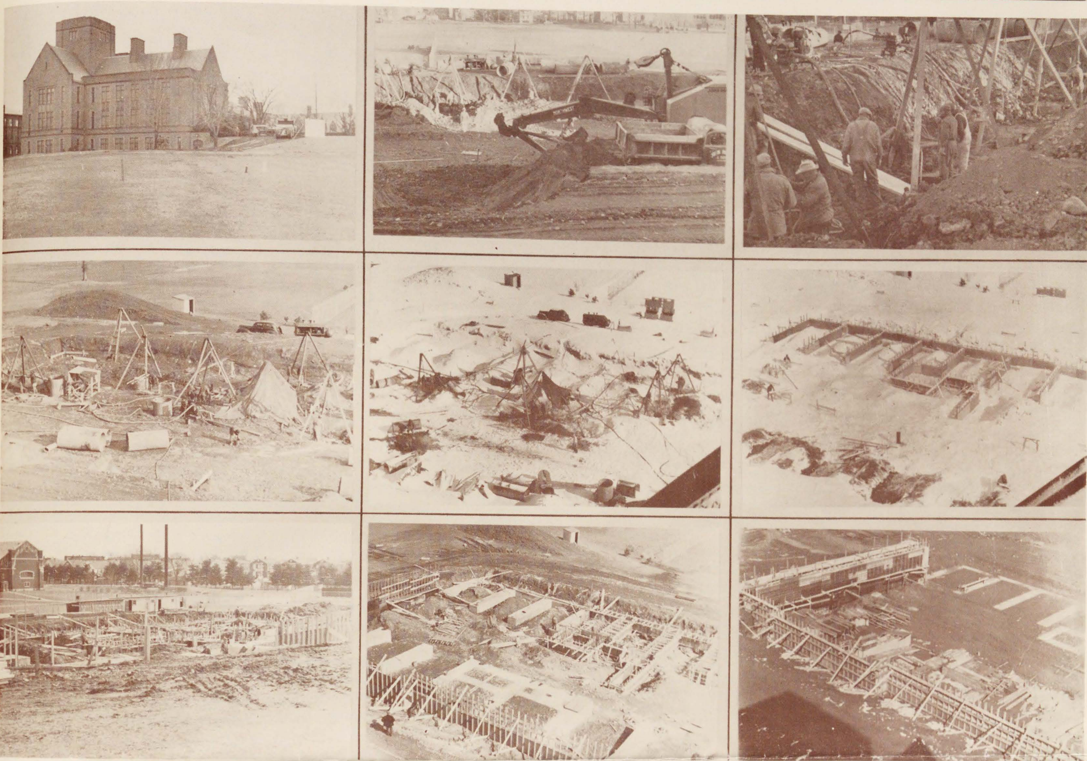
Top: Nov. 21, 1950—First day of operations; Dec. 6—Excavating for the basement; Dec. 6—Men work on the caissons for the foundation. Second row: Dec. 18—Sinking caissons is slow work; Jan. 8, 1951—Work goes on despite several inches of snow; Feb. 9—The first foundation walls appear. Bottom: Feb. 26—The work approaches the ground level; Feb. 26—The work from above; Mar. 5—The walls begin to rise.
