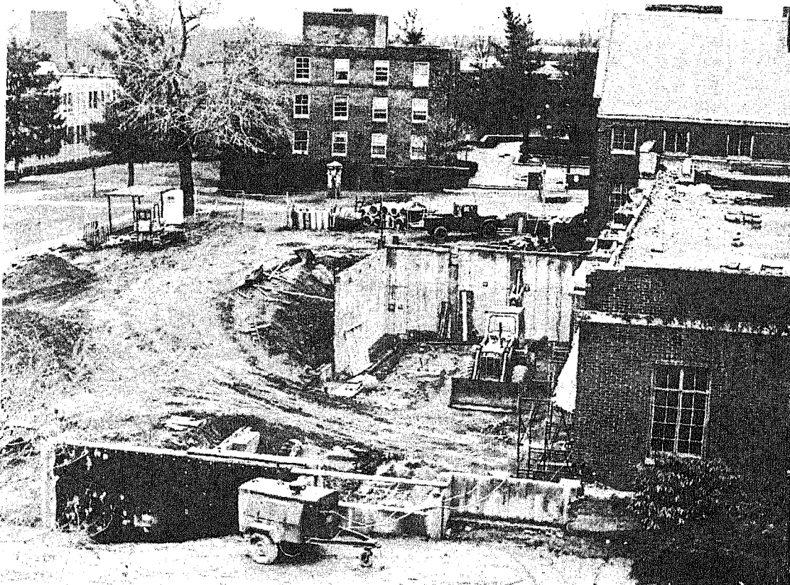
The Pit: Foundation walls begin to rise.
