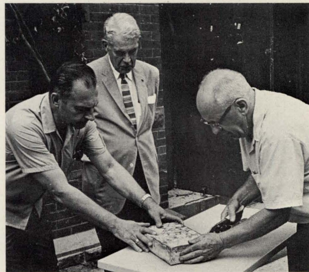
Dennis P. Tinsley, chief plant engineer, and President Jacobs watch as Walter E. Carlson, director of Buildings and Grounds carefully snips at the cover of the tin box after its removal from the cornerstone in Alumni Hall.
