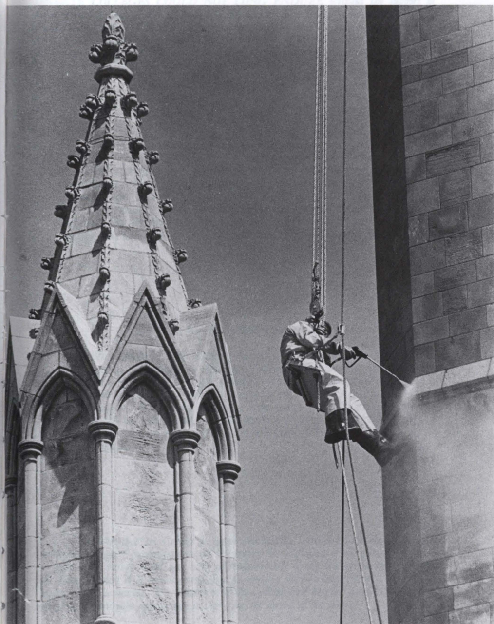
THE CHAPEL EXTERIOR received its first thorough cleaning, by high pressure water, since its completion in 1932. The Chapel's ivy and Virginia creeper vines, which had damaged its limestone surface, were also removed.
