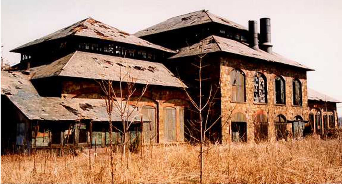
Foundry Building before renovations (Courtesy of Carnevale Eustis Architects) 87
