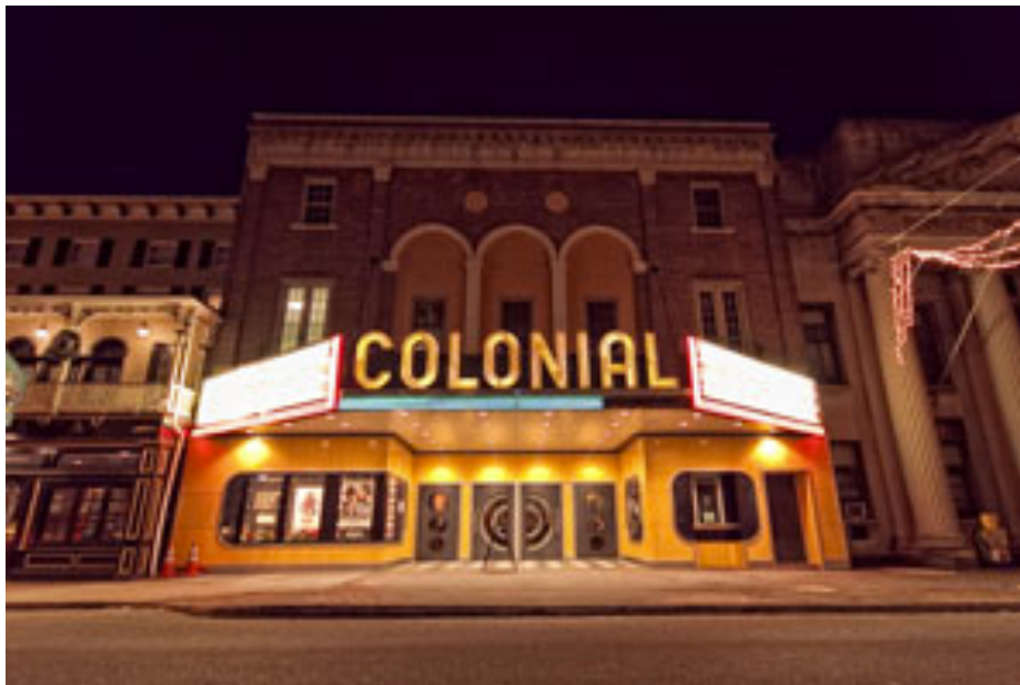
Current Colonial Theater Façade (Courtesy of Colonial Theater website)
