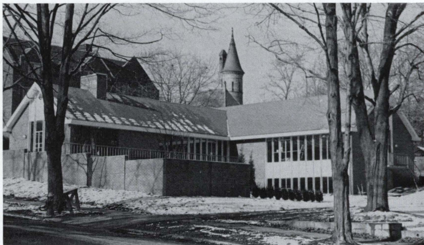
The new Alpha Delta Phi house under construction
