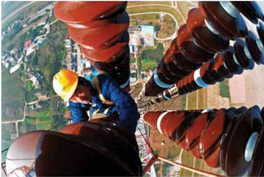
Photo 2: High on an Electricity Pylon in Eastern China
