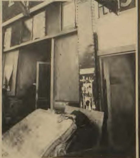
8 PANTHERS DEFENDED THEMSELVES AND THE COMMUNITY FROM 400 FASCIST STORM TROOPERS FOR 5 HOURS, FROM THIS OFFICE.
