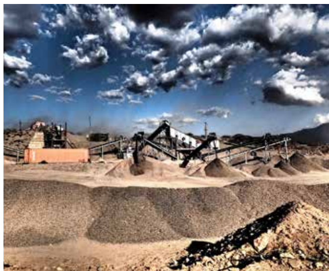
Chinese construction site, Ethiopia Photo courtesy: Sarah Tz https://flic.kr/p/rmQRuf
